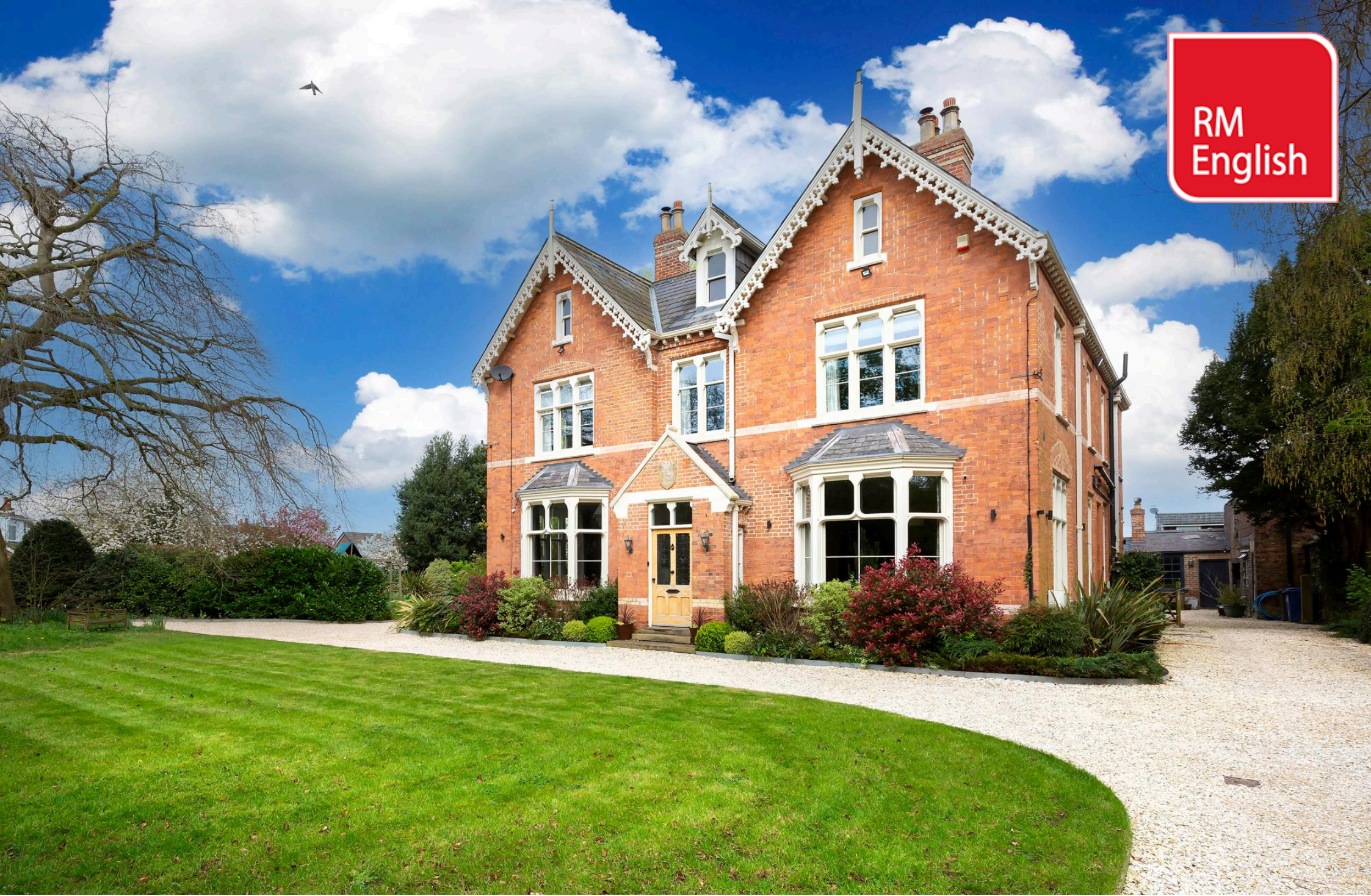
THE GRANGE, MILL LANE, CARLTON, DN14 9NG
