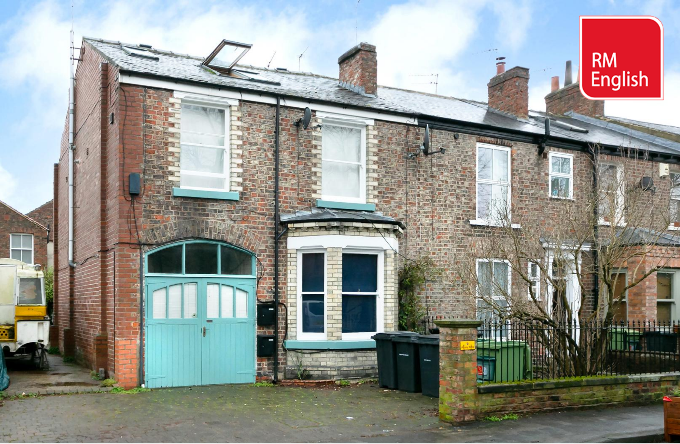
Penleys Grove Street, York, North Yorkshire, YO31 7PW
